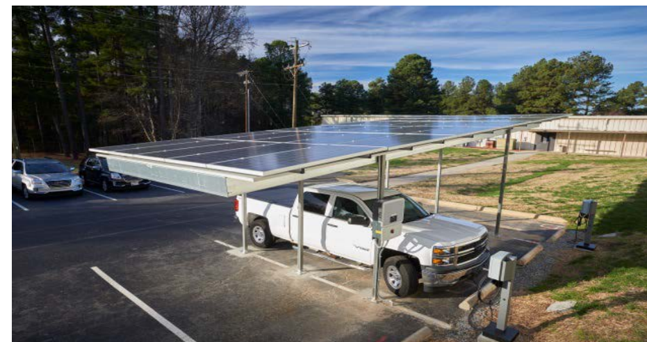
EV Carport with Rooftop Solar PV
