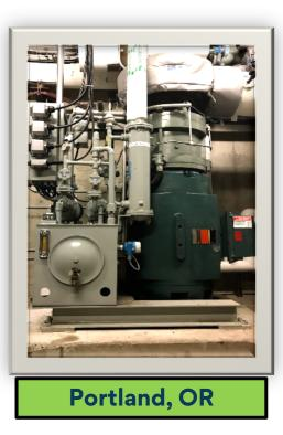
Split skid – turbine package only (controls & switchgear located locally)
