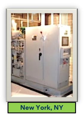
Single skid – turbine package, controls & switchgear mounted on skid
