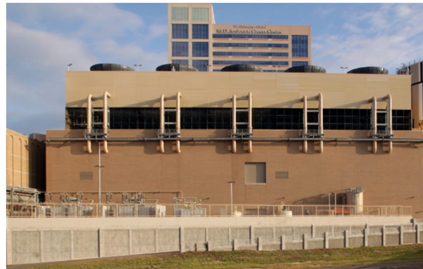
East Chiller Building 80,000 tons of capacity 32,000 tons installed
