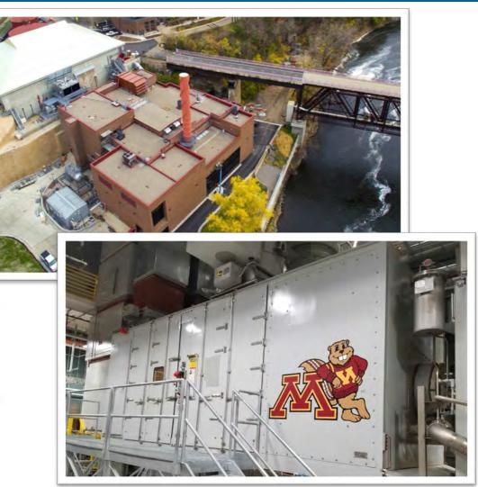
GE LM2500 DLE Dual Fuel 220 MMBtu/hr Input (HHV) 24 MWe Generator Output
