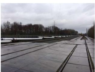
rigid steel pipe (2000 ft), induction welded joints
