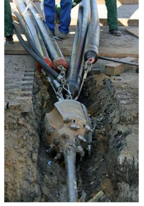
A bundle of pipes was installed in one go:
