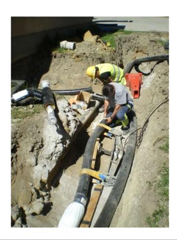
We use "flexible" pipes (stainless steel and plastic)
