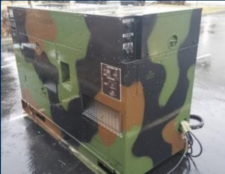
TQG before refurbishing
