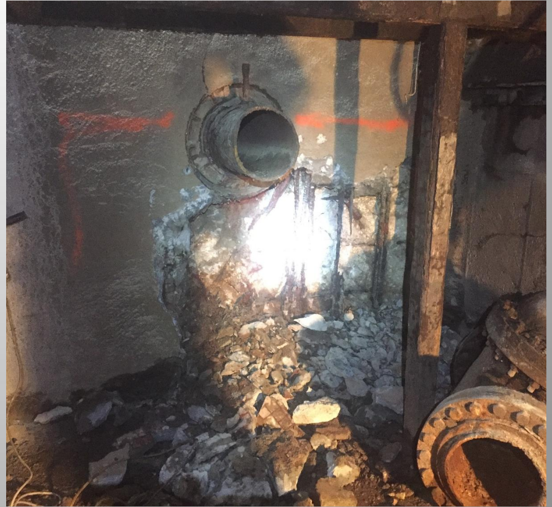
Manhole 25 wall repairs
