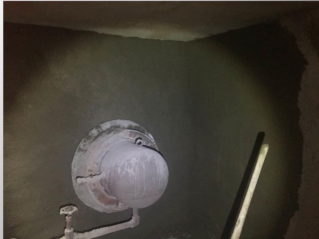
Shotcrete repair complete in Manhole 5
