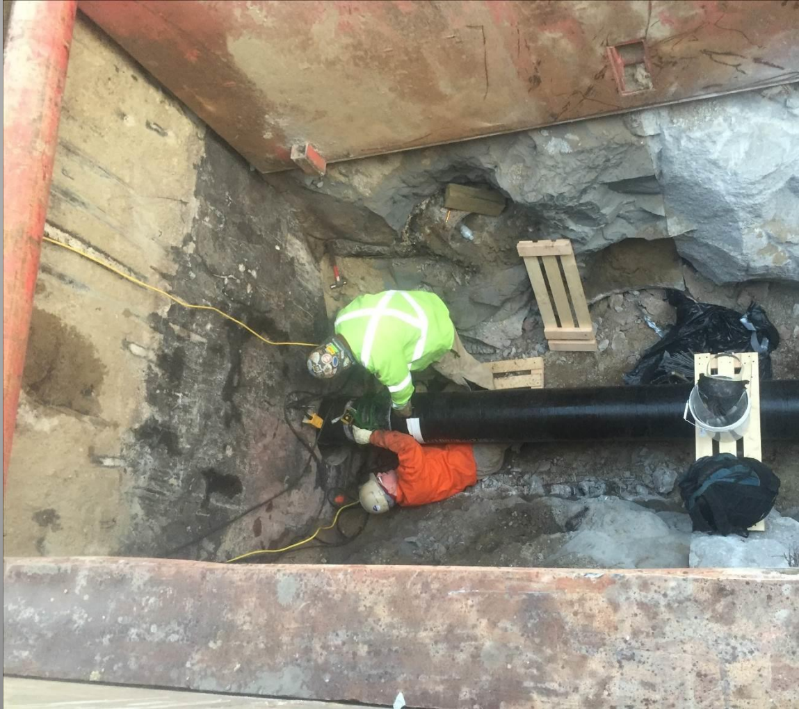
Pipe being welded in excavation east of MH 25
