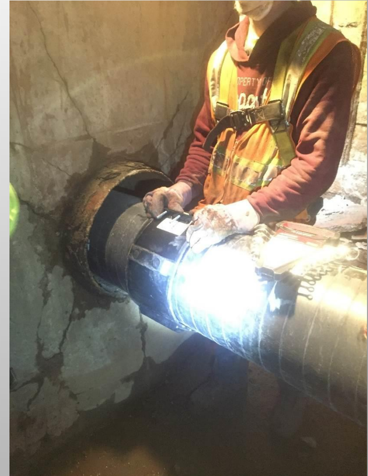
Guides being installed on new 10" pipe inside of MH 25
