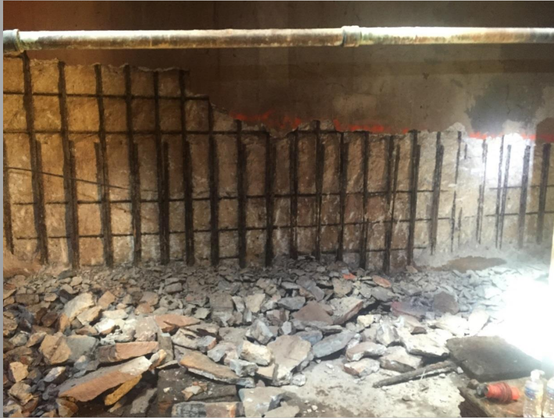
Manhole 25 wall repair started by removing compromised concrete
