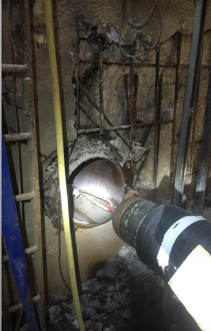
Cable pulling 10" pipe into existing 20" pipe
