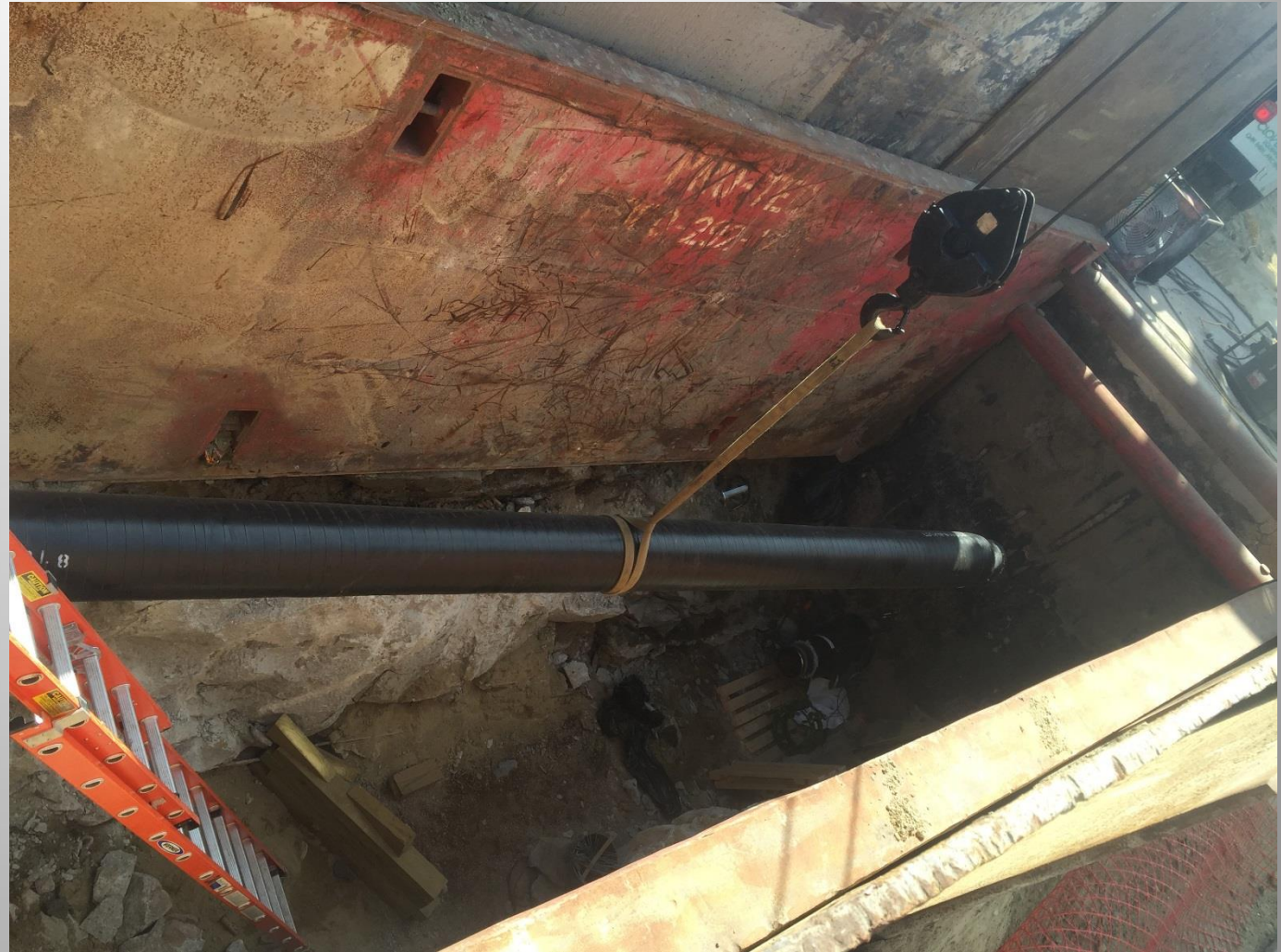
Installing Pipe in Excavation West of Manhole 5
