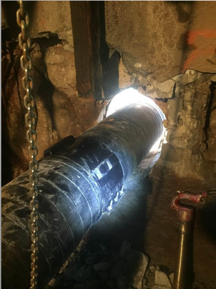
New 10" pipe is inserted from Excavation East of MH 25 into MH 25
