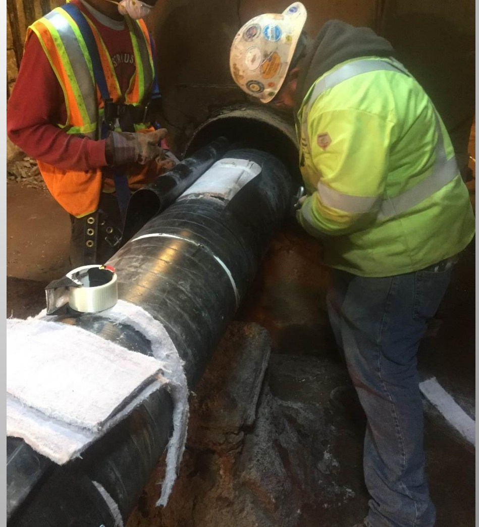
Installing Insulation kit on newly welded pipe in Manhole 25
