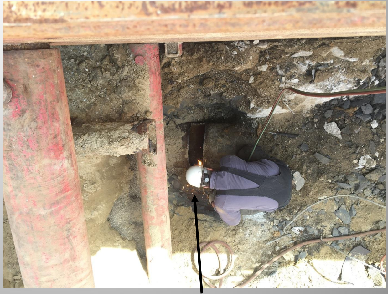
Cutting existing 20" pipe
