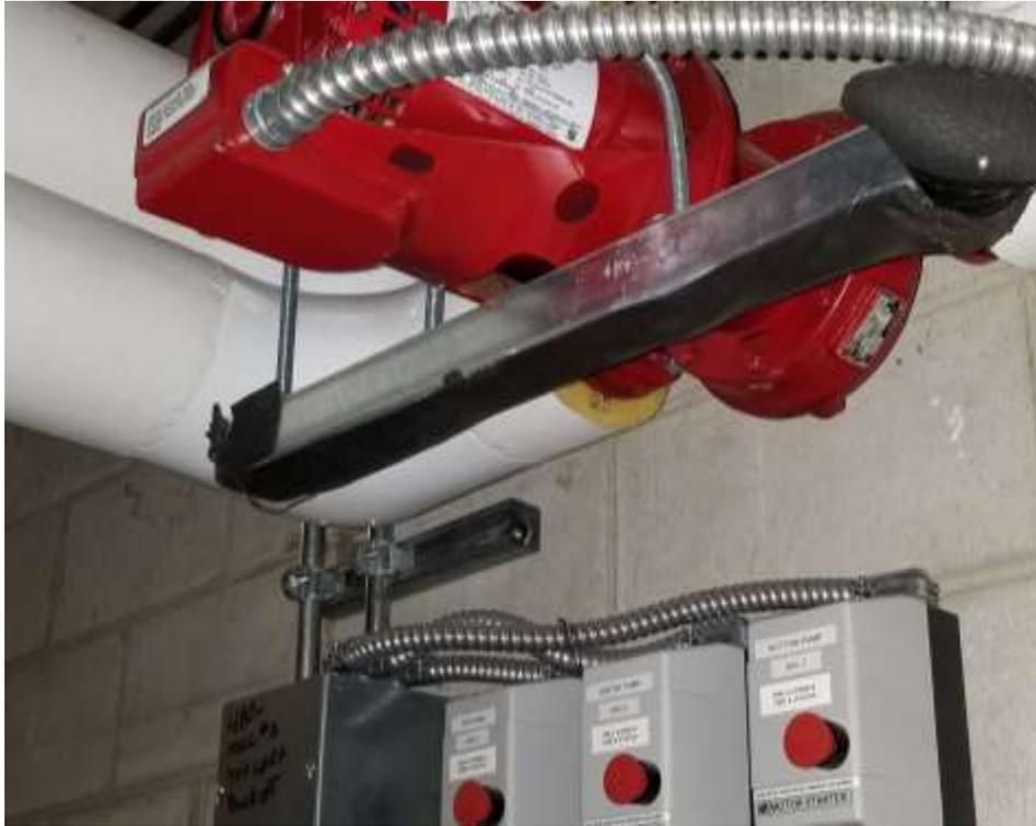
Air handler improvements to reduce preheat use included these freeze protection pumps on chilled water coils.
