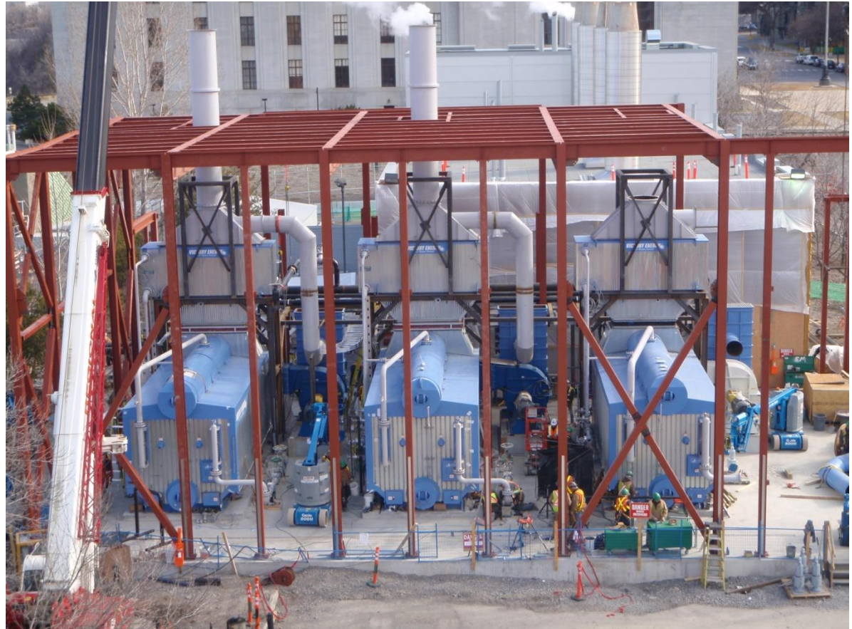
Installation of the steam boilers
