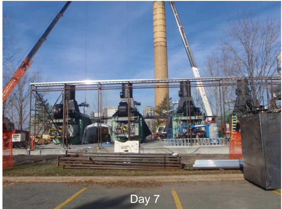
Day 7: Installation of saturated steam boilers on the concrete slab while constructing the remaining portion of the plant
