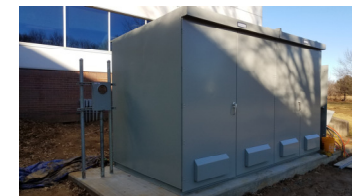
Transfer Switches (for islanding)
