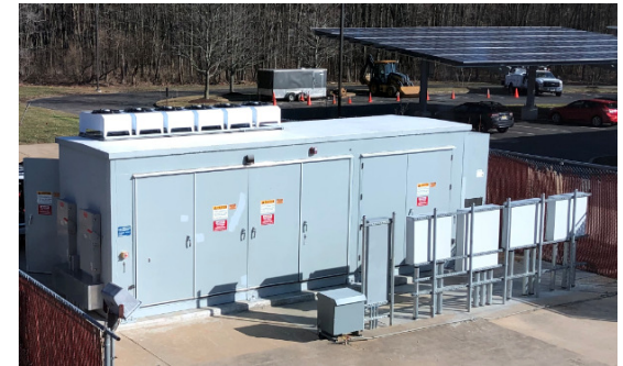
E-house (Batteries, inverters)
