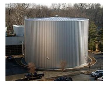
2.6 million gallon chilled water thermal Energy Storage - 40,000 Tonhour capacity
