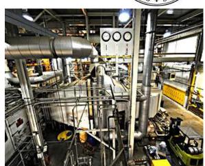
15 Mw GE LM1600 combustion Turbine 50,000 LB steam Heat Recovery, 182,000 LB with duct Burning 300,000 lb steam Boiler Capacity
