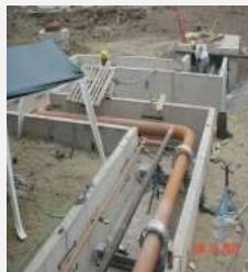
New steam piping laid in pre-cast metal insulating jacket and supported by concrete piers.
