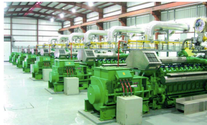
→ GENERATING ELECTRICITY WITH MULTIPLE GAS ENGINES OFFERS THE ADDED BENEFIT OF COMBINED RELIABILITY AND AVAILABILITY
