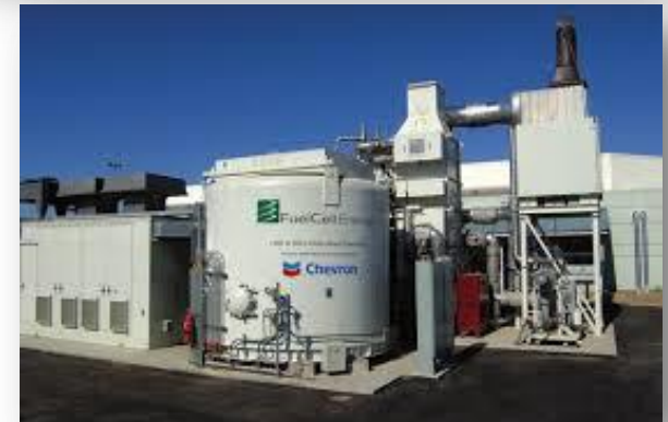
1.4 MW fuel cell plant operating on natural gas providing electricity and heat to Santa Rita Jail, County of Alameda
