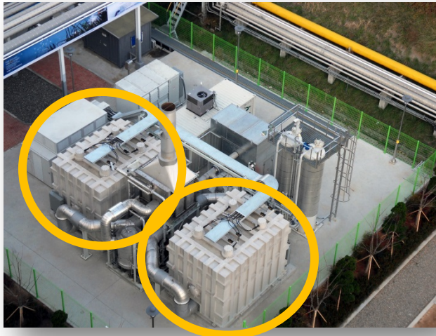
Two modules are used for a 2.8 MW power plant
