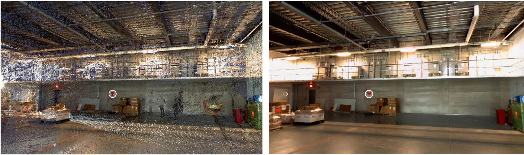
Figure – Electrical Panels on Walkable Ceiling - Laser Scan (Left) and Photograph (Right)
