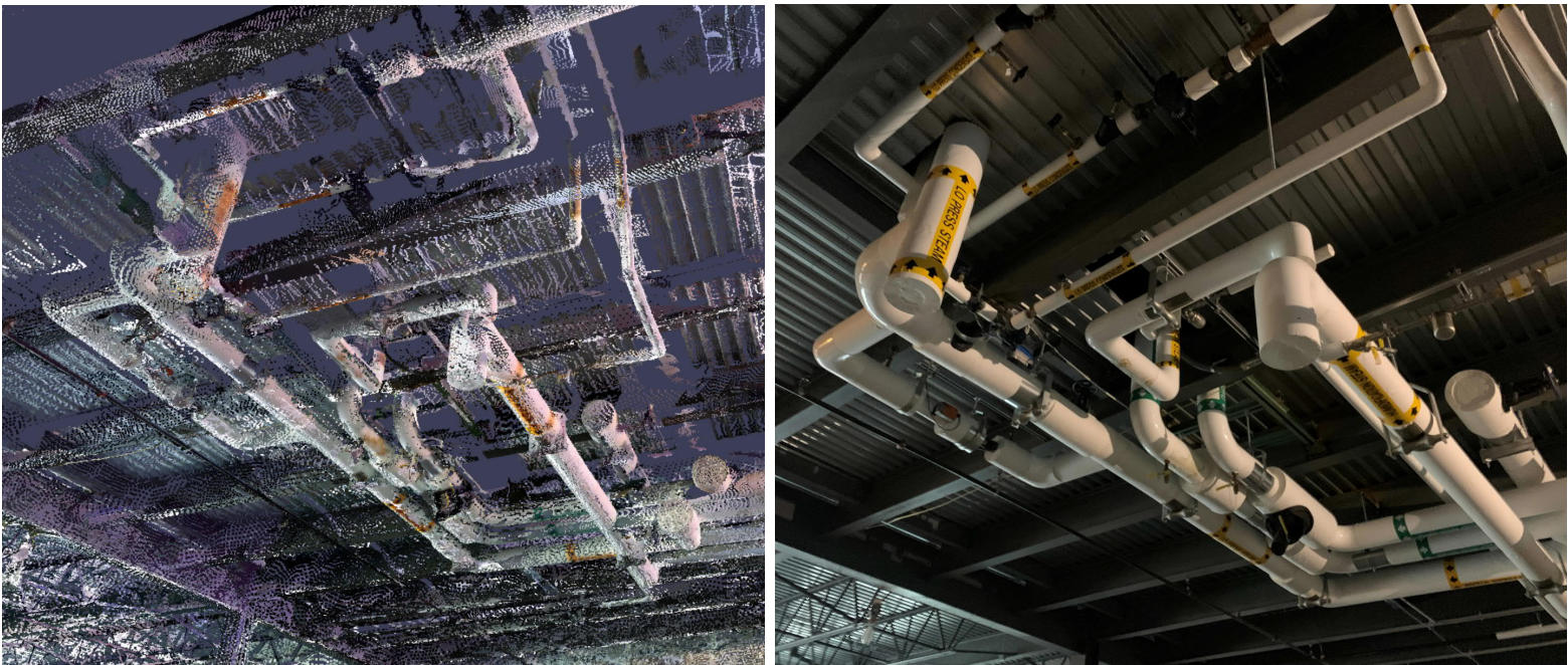
Figure – Chilled Water Piping - Laser Scan (Left) and Photograph (Right)
