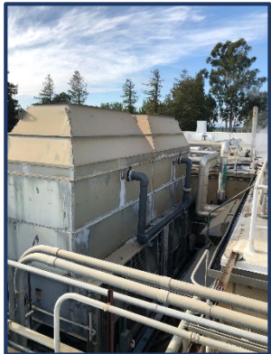
Cooling Tower Poor condition
