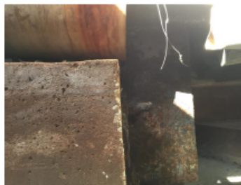
Rusted and Broken Anchor Plate on 6" 70S
