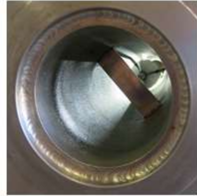
Fig 2. Inlet View of a VorCone Meter
