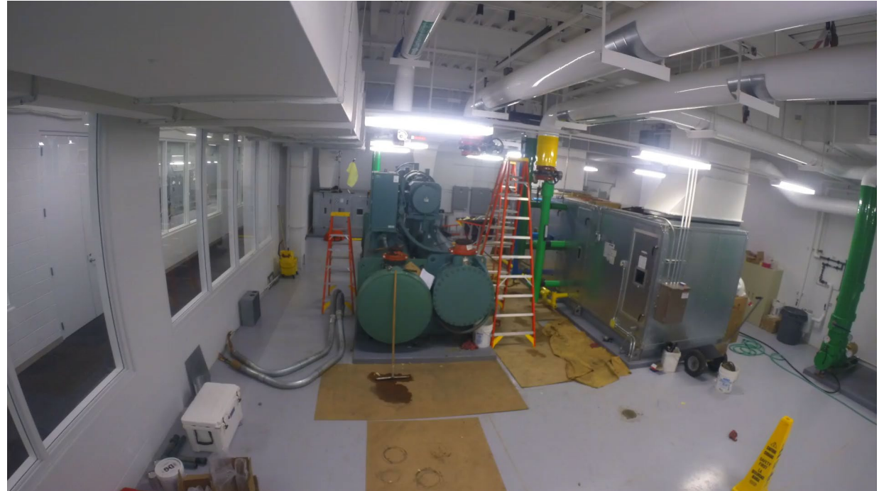
Replaced oil bearing centrifugal chiller
