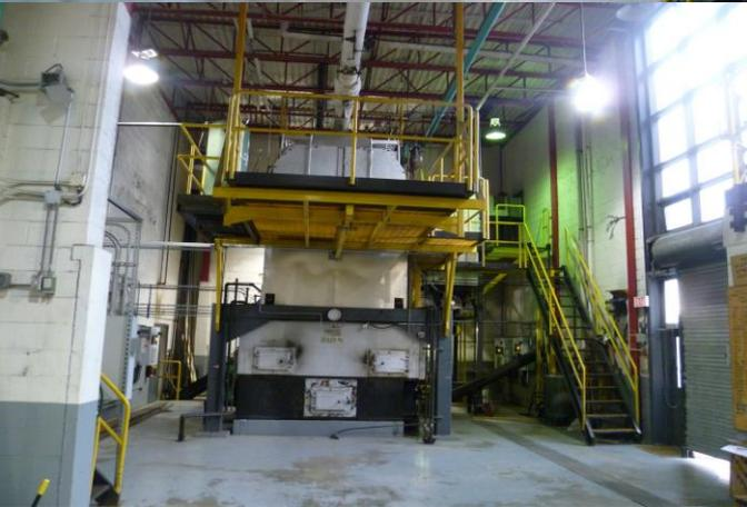
Boiler # 3 – 12,000 pph, HP steam boiler (furnace oil), 36 yrs old
