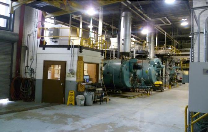
Boiler #1 – 20,000 pph, HP steam boiler (furnace oil), 48 yrs old
