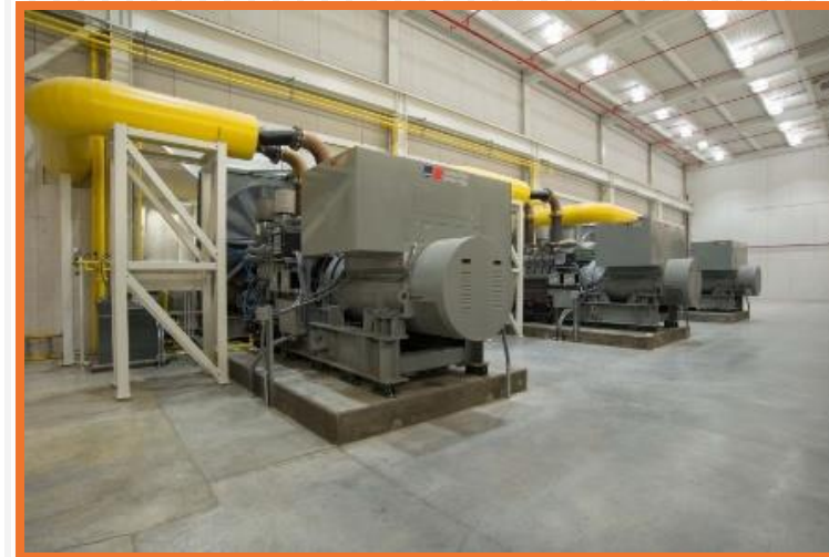
N+1 Back-up Generators for ADF and Plant – 5.4 MW
