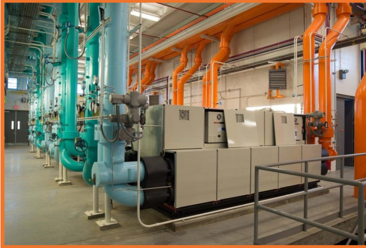
Nominal 300 ton Scroll Heat Pump Banks
