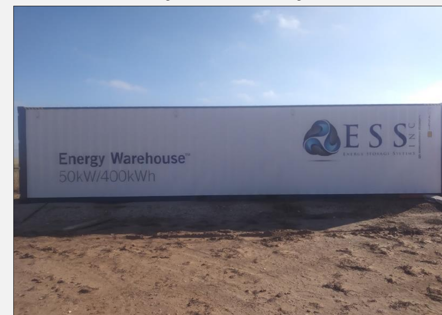
Figure 10: 50 kW battery
