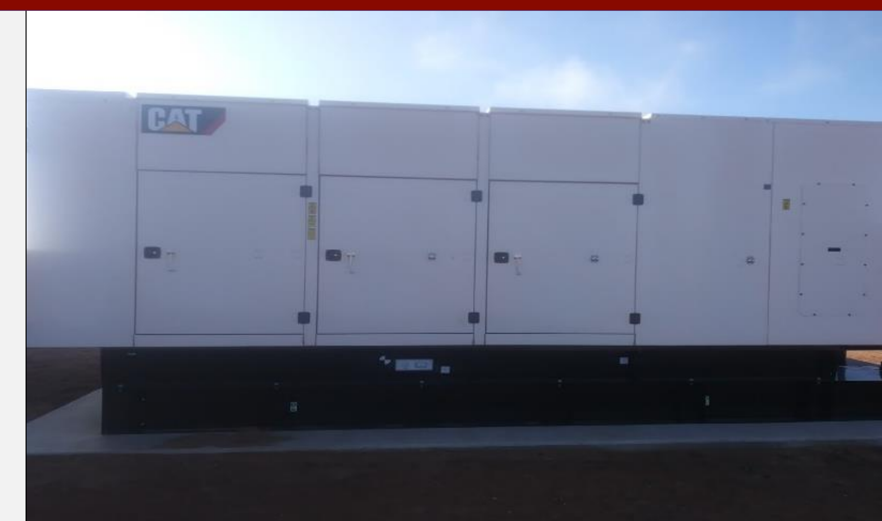
Figure 7: Tier 4 diesel generator
