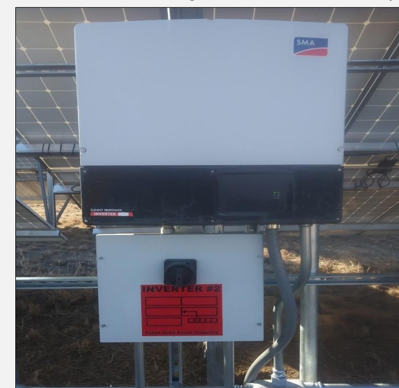
Figure 8: 30 kW solar inverter
