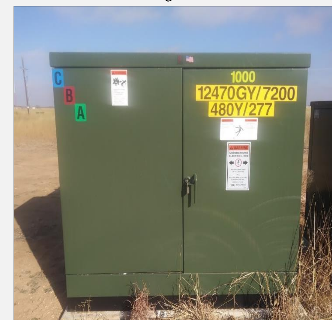
Figure 9: Step up transformer
