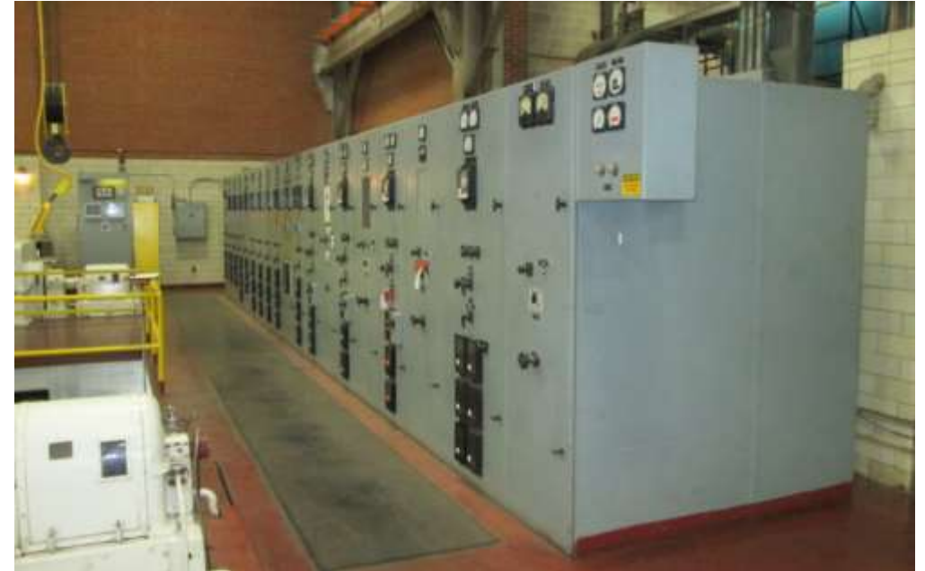
Old switchgear lineup in Power Plant
