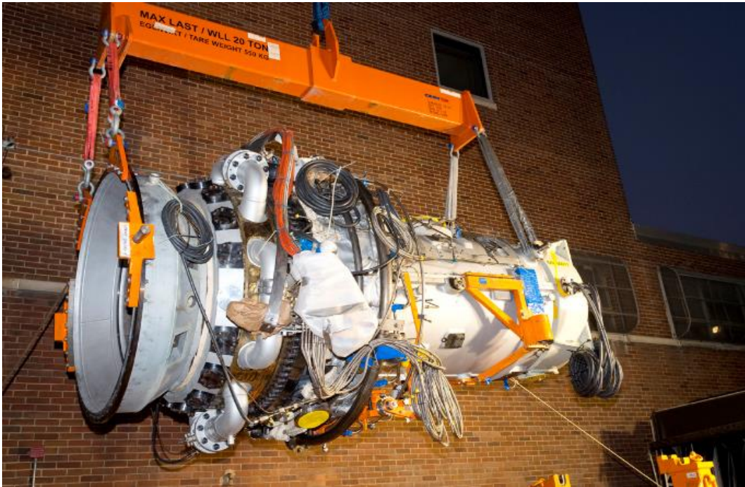
CHP plant at National Institutes of Health (Maryland, US) SGT-600 Gas Turbine 23 MW(e) and heat requirements on campus
