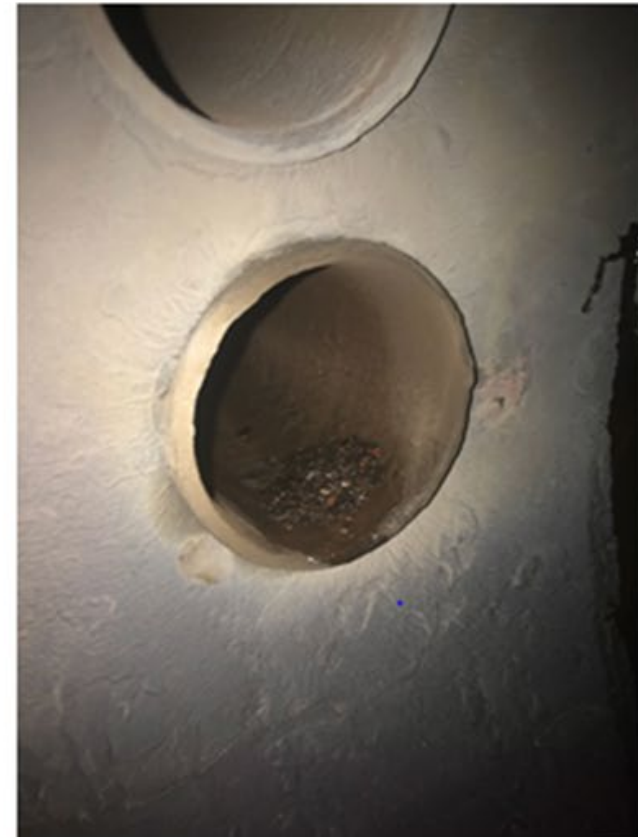
2018 Inspection - Mud Drum Third Row Tube
