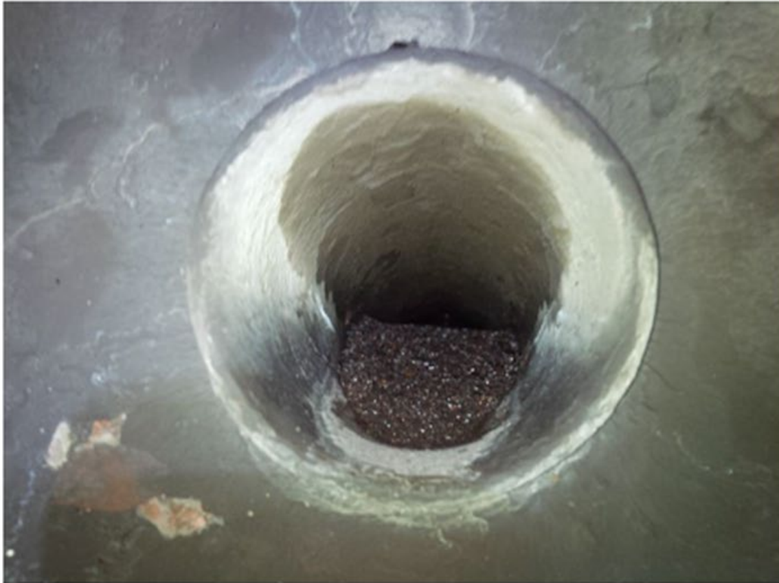
2015 Inspection - Mud Drum Third Row Tube
