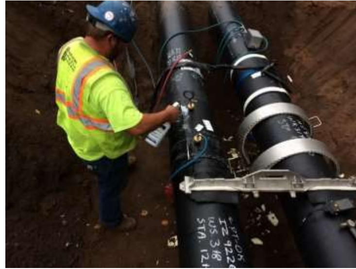
Testing All Joints
