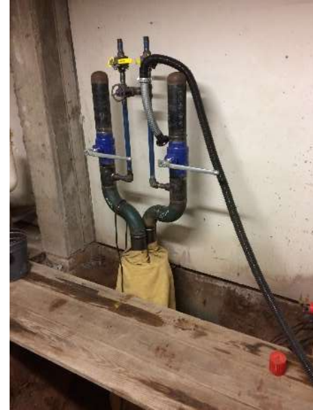
Twin Pipe Customer Connection
