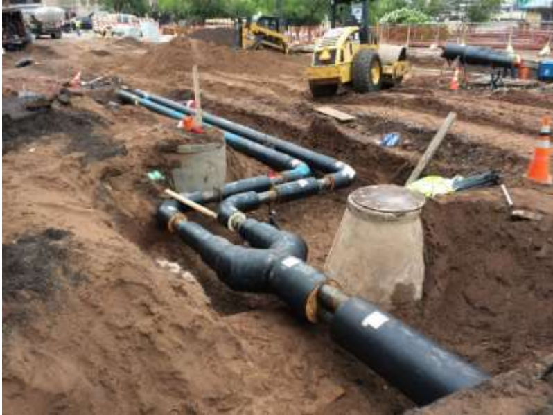
Twin-Pipe Connection
