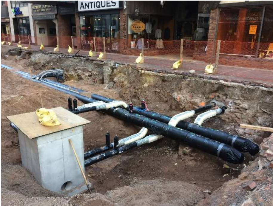
Direct Bury Valves/Drains/Vents
