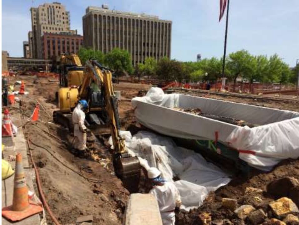
Existing Steam Pipe Asbestos Abatement
