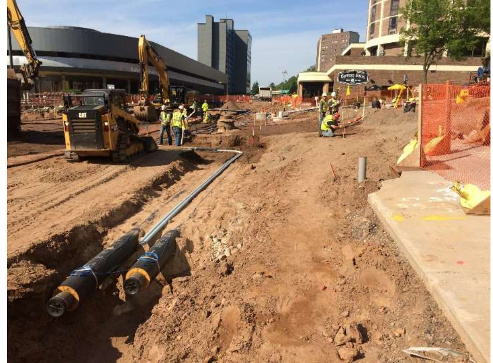
Hot Water Distribution Construction
